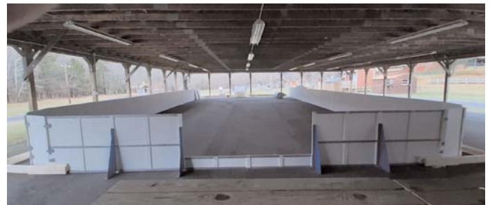
Our ICE RINK construction in progress. Looking good!
