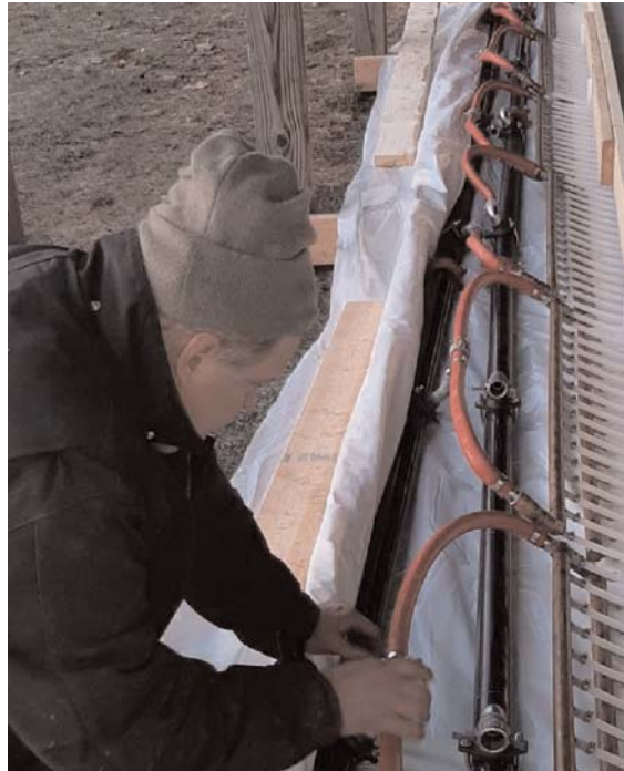
Ric Coombe checking the connections
