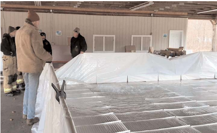
The Neversink Fire Dept spraying in the water to form the first layer of the ice
