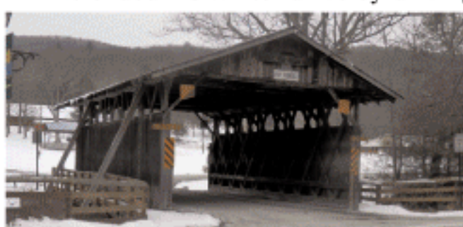
Bridge at the entrance of the fairgrounds
