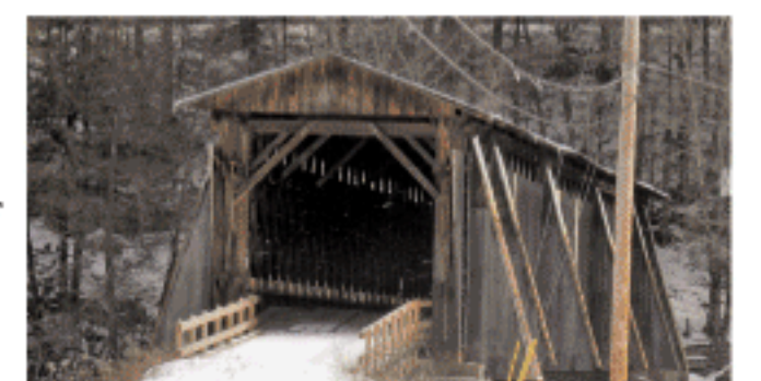
Halls Mills Bridge
