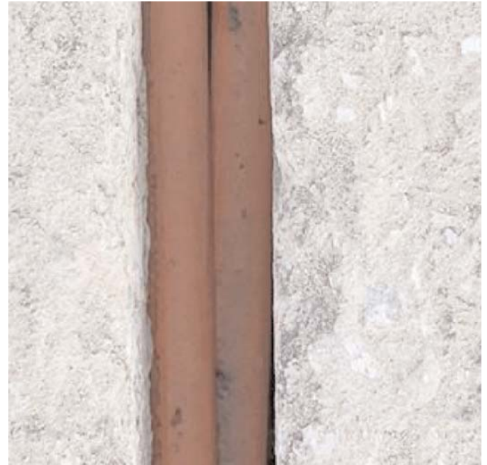
The fiber-optic conduits sit snugly inside the microtrench.
