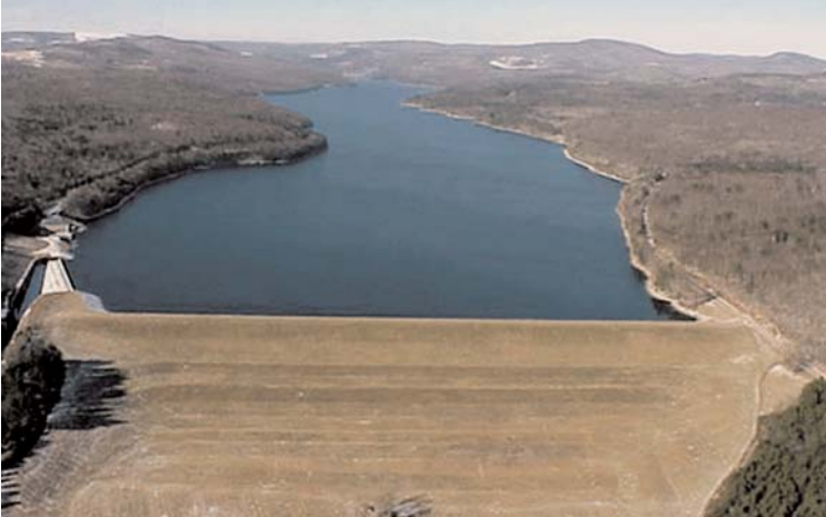
Rondout Dam Valley
